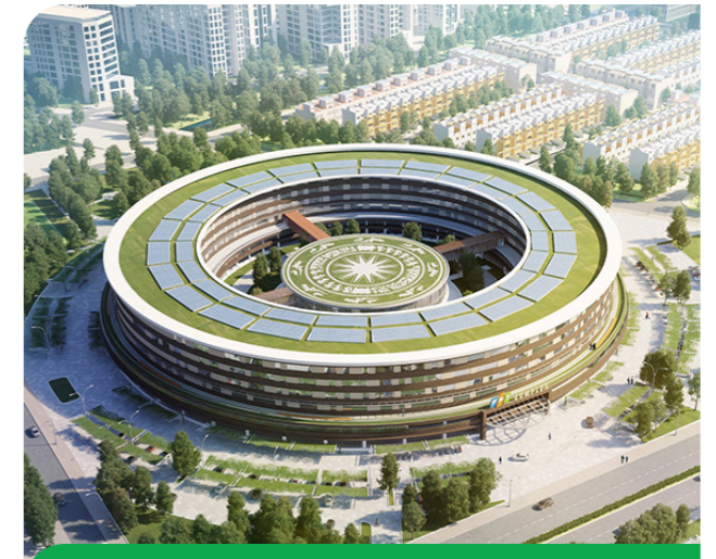
FPT Complex Da Nang is the first building in Vietnam to achieve the EDGE certification, thanks to solutions such as energy efficiency, rainwater harvesting, wastewater treatment, and high-efficiency air conditioning and lighting systems.
