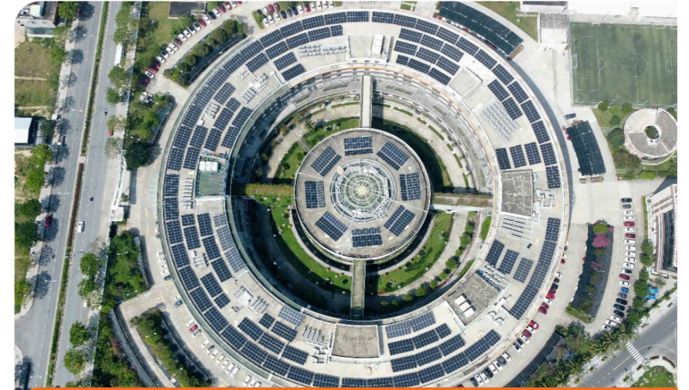
Rooftop solar power system at FPT's campus in Da Nang.
