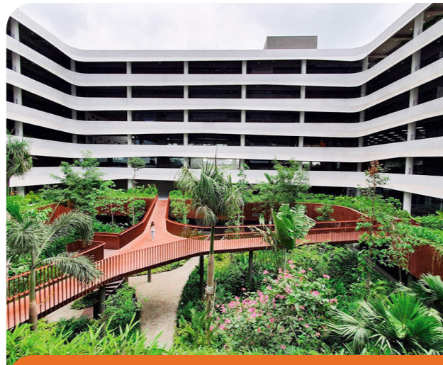
F-Town 3 was recognized by Wallpaper, a leading architecture and design magazine in the United Kingdom, as a representative project of bioclimatic architecture, where more than 40% of the space does not require air conditioning.
