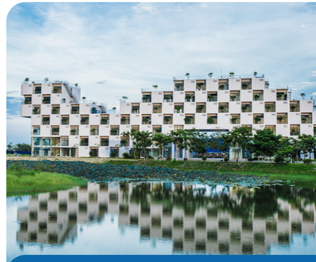
The FPT Administration Building in Hoa Lac was honored at the World Architecture Festival in the Future Education category and received the First Prize for Green Architecture awarded by the Vietnam Association of Architects.
